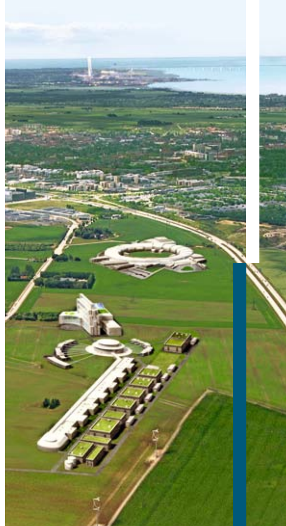
Construction of the planned European Spallation Source in Lund. The ion source at the front of the picture generates the proton pulses, which can be accelerated to almost ninety percent of the speed of light. The round part of the building houses the target. It contains a heavy metal, such as lead or mercury. The collision between the protons and the metal atoms charges the atoms energetically, causing between twenty and thirty neutrons per atom to “vaporize”. These are then decelerated and directed onto the specimen to be examined. The inner structure of the sample material is then reconstructed based on the way in which the neutrons interact with the specimen being examined.
